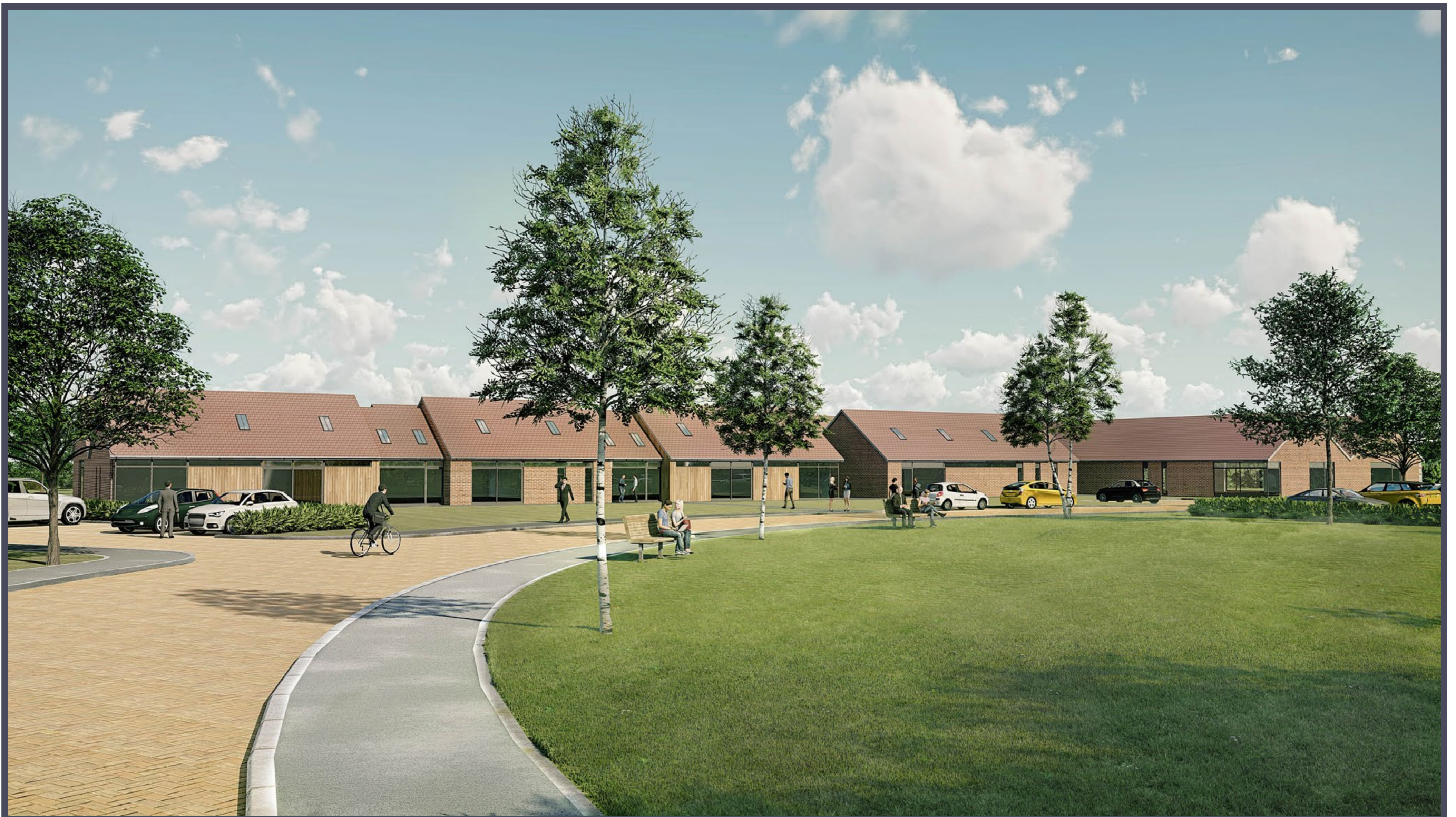
View of office buildings from site access
